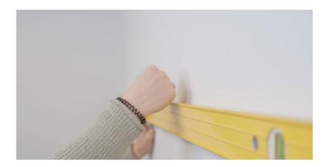
**Step 2:** Screw the back clips to the wall making sure they are touching and are level with your line across the top.
