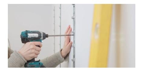
**Note:** If fixing into timber studs screw through the top hole of clip but not all the way in. Ensure the back clip is level vertically and then tighten screw and repeat on bottom hole on the back clip. For maximum holding capacity ensure you fix a screw in every hole of back clip.
