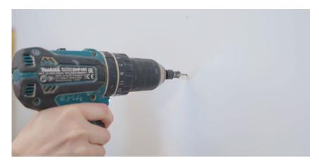
**Step 7:** Place your FlexiTrack strip back up on the wall and fix using the white headed screws provided. Be careful not to overtighten.
