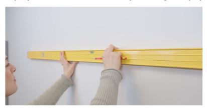
**Step 3:** Using your pencil, make some marks on your FlexiTrack strip to indicate where you want the screws to be placed. For optimal results, we recommend spacing the screws evenly along the strip, ensuring that you place one screw at each end, approximately 5-10cm from the edges.
