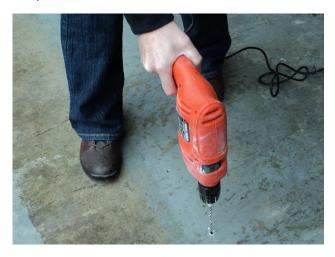
Remove the Threshold Seal and using a 6mm masonry drill bit, drill holes in to the floor where you have marked the ground. (Drill holes are spaced approximately every 200mm and 50mm from each end).
