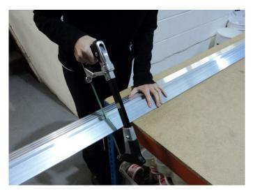
Cut the end aluminium sections to size / shape and cut the two bottom rubber seals and the top cap to the required size.
