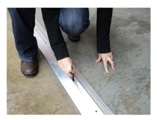
(**Position A**) Position the Threshold Seal in line with the centre of the door so the door will close on the black and yellow cap that runs along the centre of the aluminum section(s).
