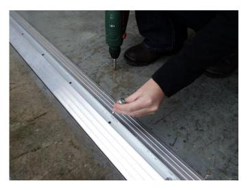
Apply pressure on the Threshold Seal by standing on it. This will compress the two side seals. Then tighten the fixing fully.
